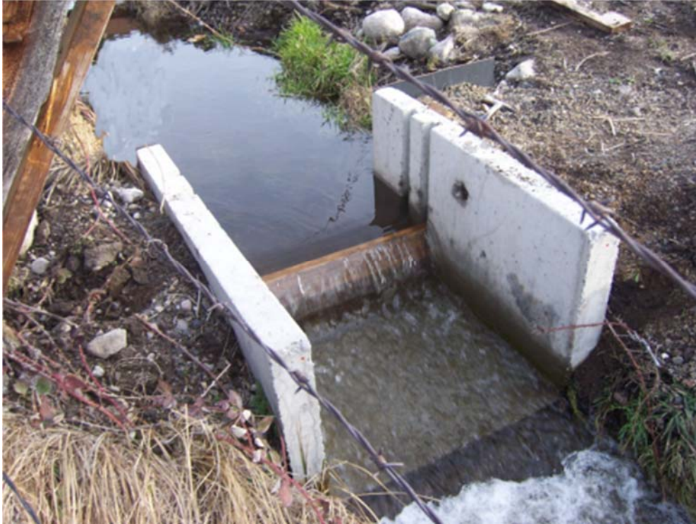
Figure 14. Example of a water control weir with flash boards.
