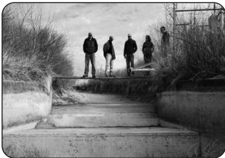
Navajo Engineering Construction Authority will complete construction on a weir wall at the Hogback Diversion Dam on the San Juan River in early 2013. The fish weir will prevent endangered fish from becoming trapped in the canal.
