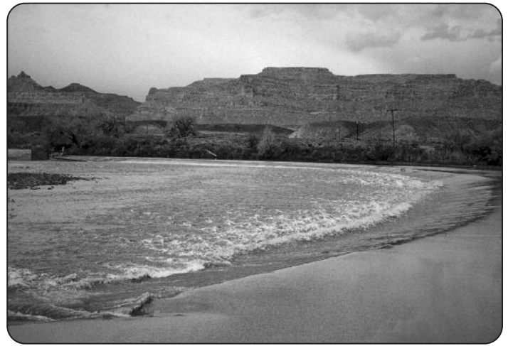
Construction of an electrical barrier at the Tusher Wash Diversion Dam and Canal in eastern Utah is the last major capital project currently identified in the recovery goals for the Upper Colorado River system.
