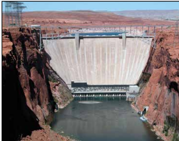
Glen Canyon Dam.
