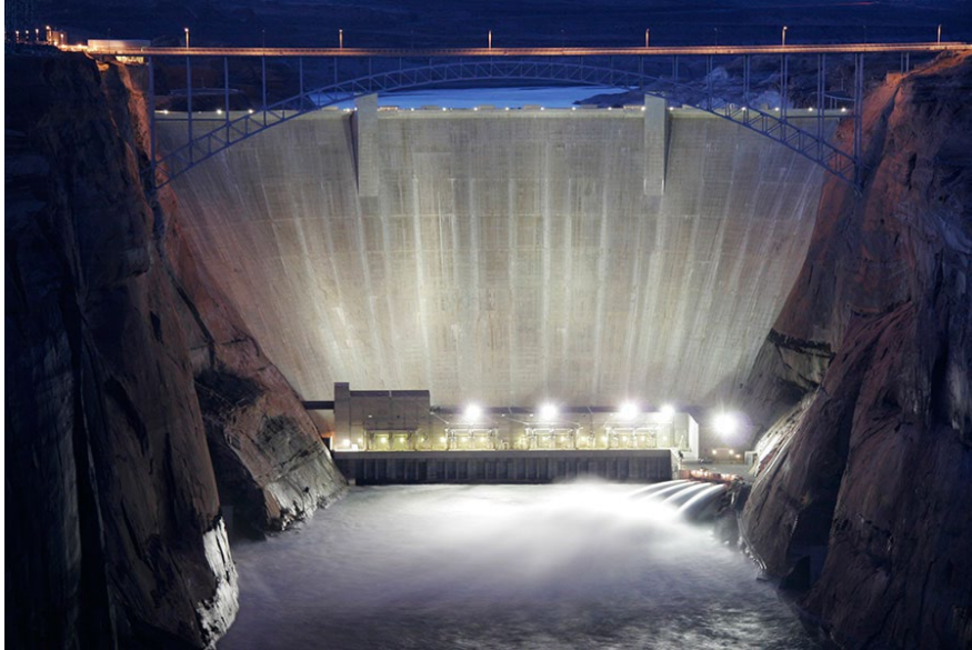
Figure 2. Photograph of Glen Canyon Dam looking upstream with powerplant at the downstream toe of the dam and four outlet works discharging at river left.
