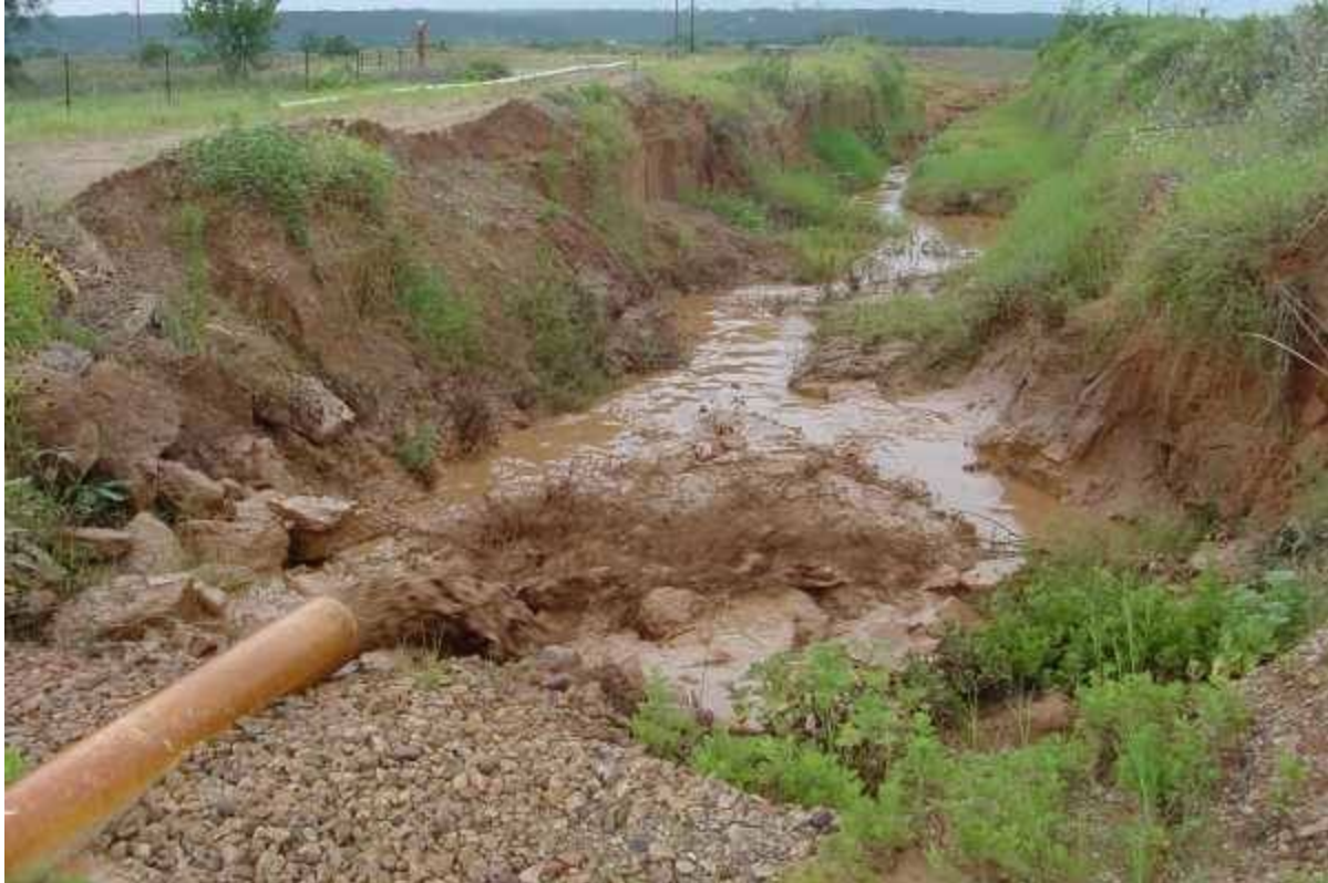
FIGURE 6 Discharge of Sand Slurry from Hydraulic Dredge System.
