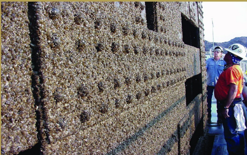
Davis Dam Penstock Gate Oct.07
