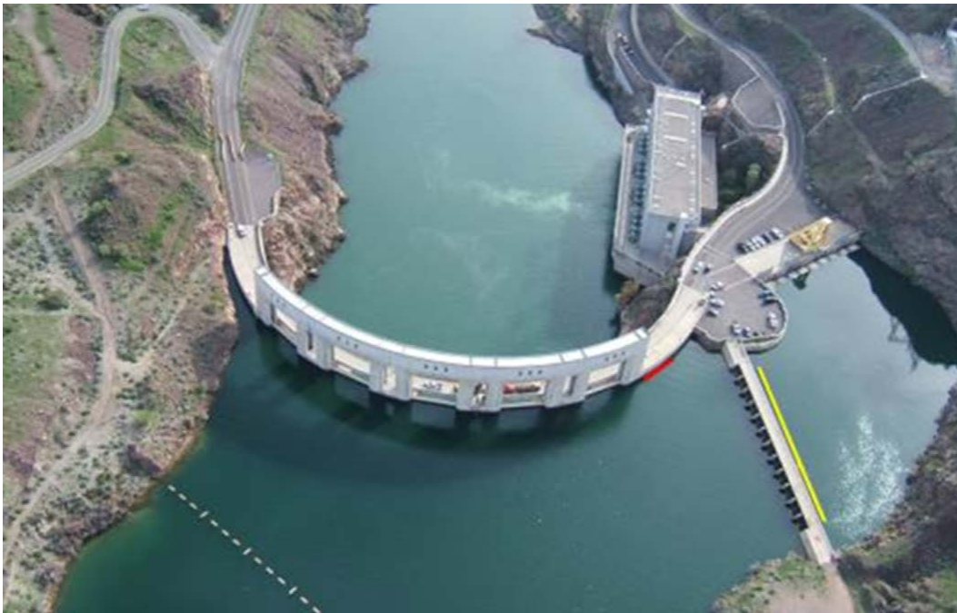
Figure 1. Aerial photo of Parker Dam, CA. The red line indicates the location where the plates were placed, and the yellow line indicates where the grates were placed.
